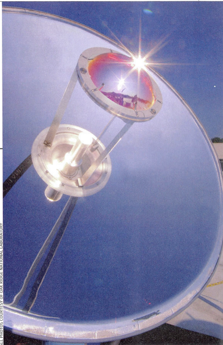
In a hybrid solar lighting system, a rooftop-mounted collector separates the sunlight's visible segments from infrared segments to generate lighting and electricity, respectively.
