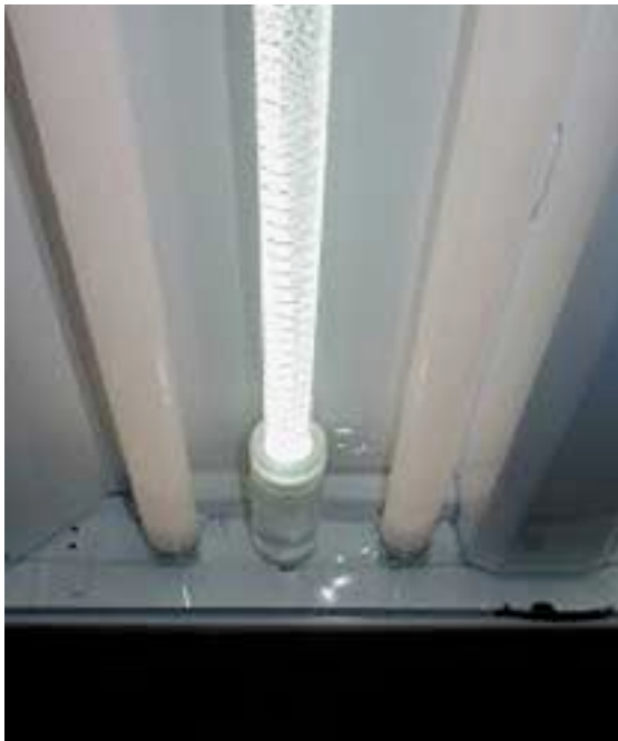
Internal view of a fluorescent hybrid luminaire. Two fluorescent lamps can be seen with a sunlight-diffusing rod between them. Photo courtesy TVA.
